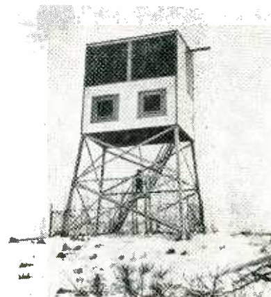
Transmitting tower for Workshop's new antenna pattern-measuring range
